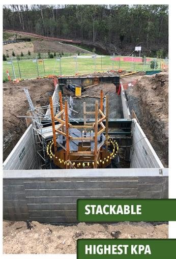
With the ability to combine an extensive range of panel and spreader sizes, our staff can design and supply the correct solution for any sized excavation. With the ability to stack boxes and provide higher pipe clearance with supporting arches, no hole is to big or to small.
